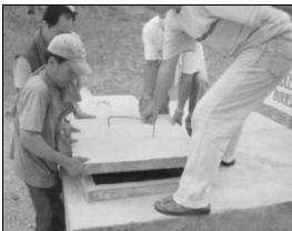
Photograph 18. Cover of a Rectangular Concrete Septic Vault
