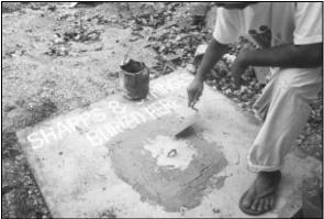
Photograph 23. Sealing of a Concrete Vault
