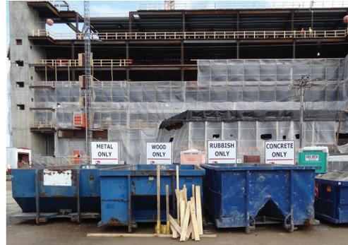
Contractors set up dumpsters at the Gundersen construction site to sort the waste materials. Since 2010, construction recycling/reuse rates for the new Hospital and Inpatient Behavioral Health Building has exceeded 93 percent.
